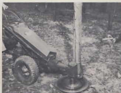
CLEAR LAND, CUT TIMBER
